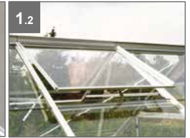
1.2 Window Exterior view
